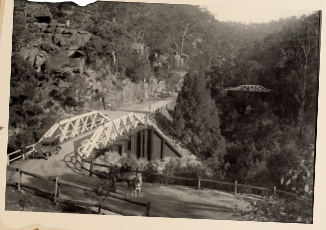
Galston Bridge, Galston Gorge
